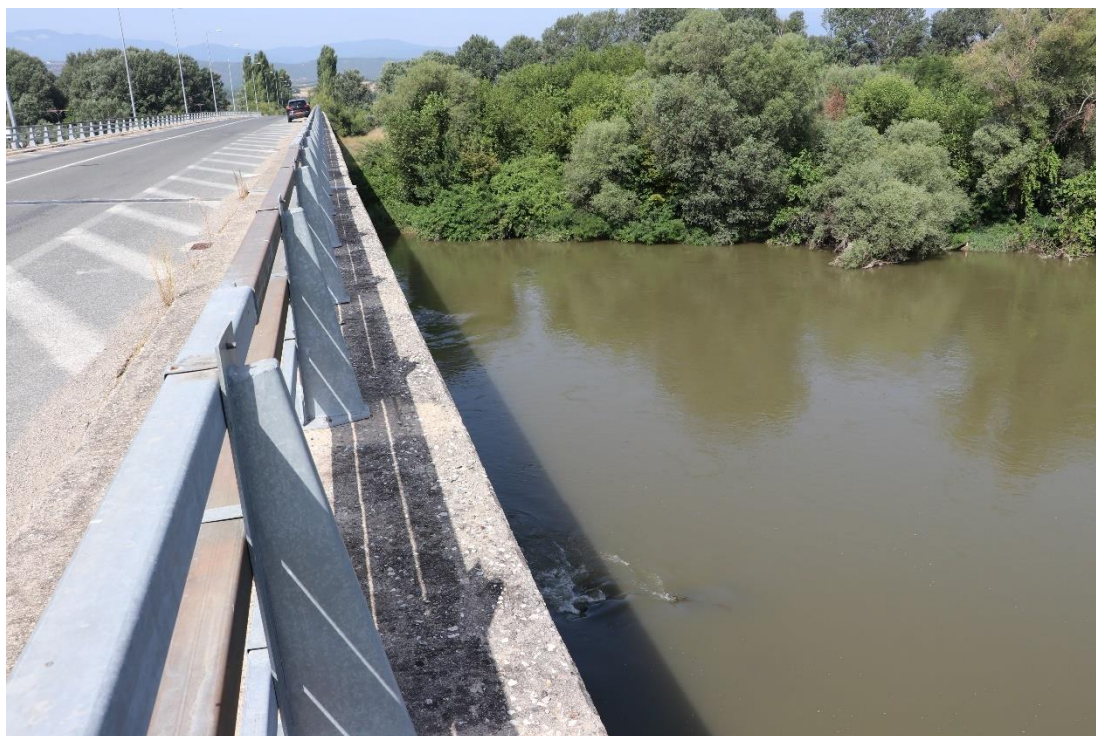
Picture 2. Photo of the installation site on the Idomeni bridge
