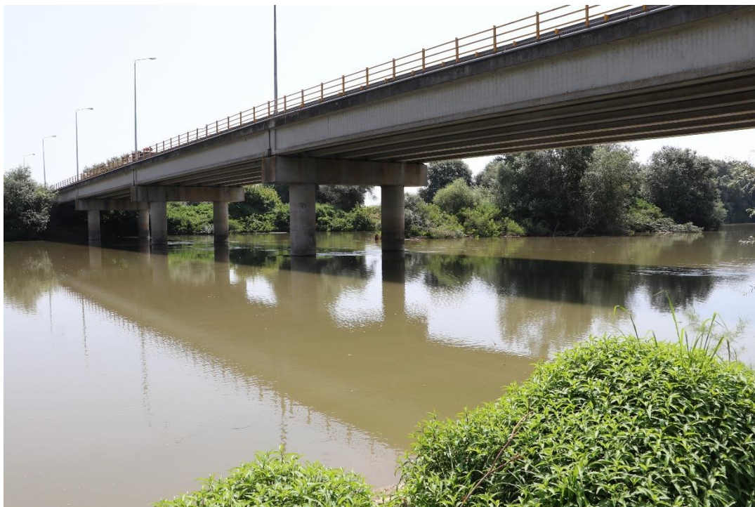
Picture 1. Photo of the installation site on the Malgara bridge
